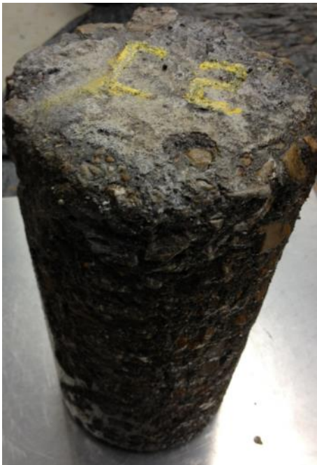
Figure 8 – Untreated Sample after 18-months showing a little more than 500grams of concrete loss
