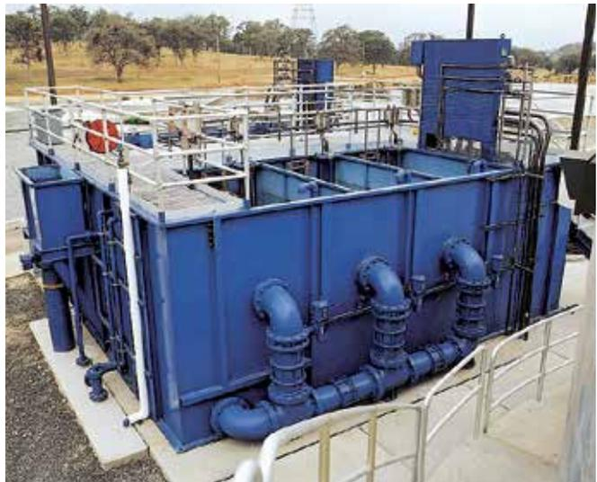
The Chem-Clean® system restores the sand to its original condition.
