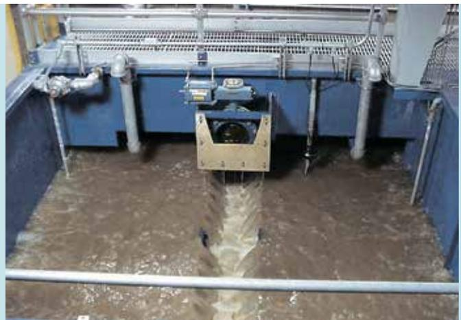
Backwash water flowing in trough, air assisted
