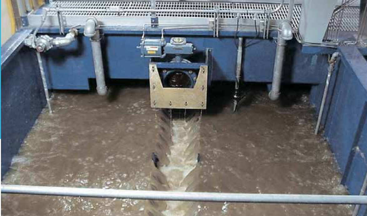
The Hydro-Clear® filter was designed specifically for filtering wastewater treatment plant effluents
