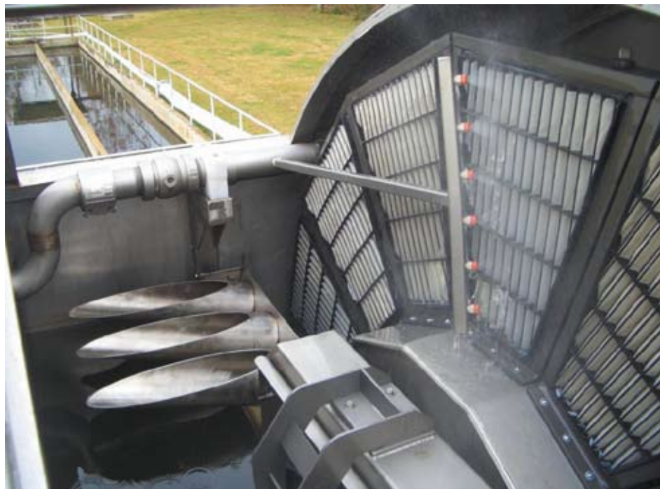
The backwash process in disc filters is initiated by headloss. High-pressure nozzle sprays dislodge accumulated solids, propelling them back towards the inside.
