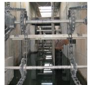
**Stub shaft:** Cast iron tripod with extendable metallic stub end to accommodate tank wall irregularities. Fabricated heavy-duty stainless steel for extreme duty.
