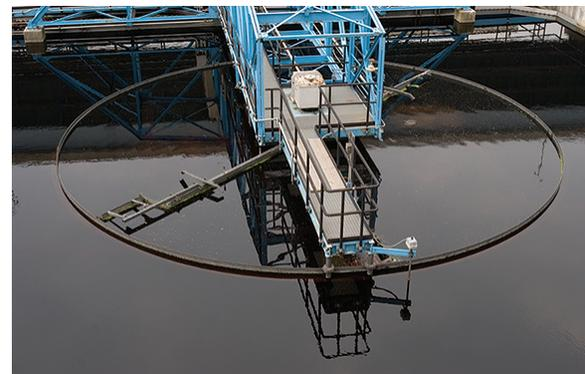
After FEDWA Baffle System settling is improved
