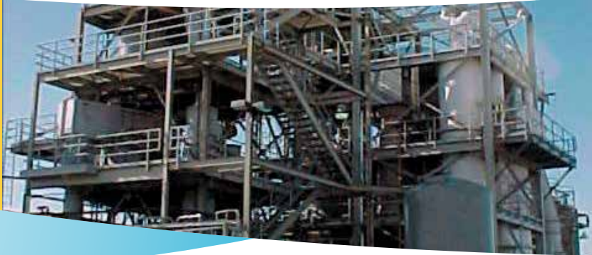
CARBON REACTIVATION FACILITY
