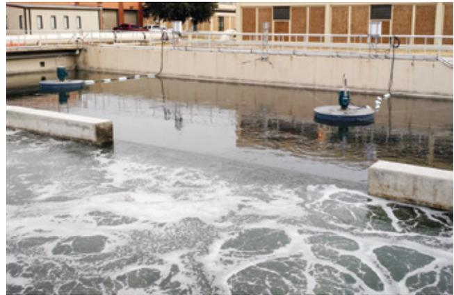
Aqua-Lator® Direct Drive Mixers are an ideal solution for anaerobic and anoxic tank mixing in wastewater treatment applications.
