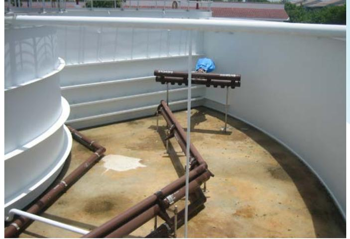
The outer diameters of all four OMNIPAC® SBR systems range from 60 to 105 feet in diameter. Each unit contains three SBR basins with jet aeration systems to mix and aerate the mixed liquor, a solids-excluding floating decanter for effluent withdrawal and an influent manifold for the even distribution of influent into the sludge blanket.
