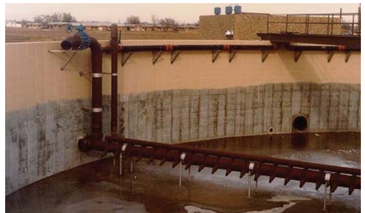
Pneumatic Backflush Cleaning System
