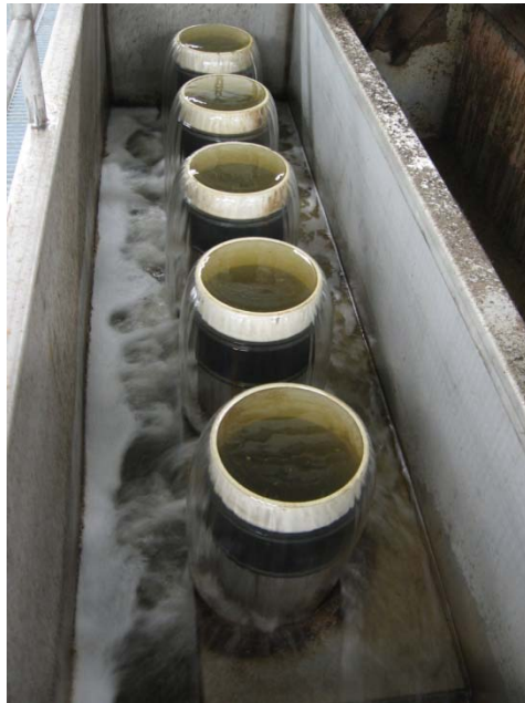
Figure 9. Effluent from DAF providing clarification of aerated tank mixed liquor
