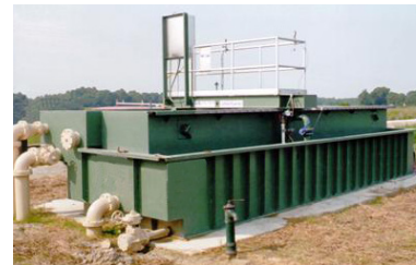
Gravisand® Traveling Bridge Filters
