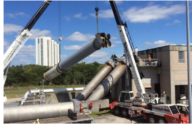
Inspect, repair or replace screw pumps
