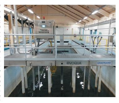
final polishing before disinfection and storage in the finished water clearwell. Each unit can operate separately or in parallel for maintenance or demand needs.
