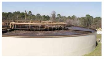
Utilities, Inc. of Longwood, FL partnered with Evoqua to rehabilitate three biological wastewater treatment trains to restore operating efficiency, extend the plant's useful life and meet capacity and nutrient removal requirements.
