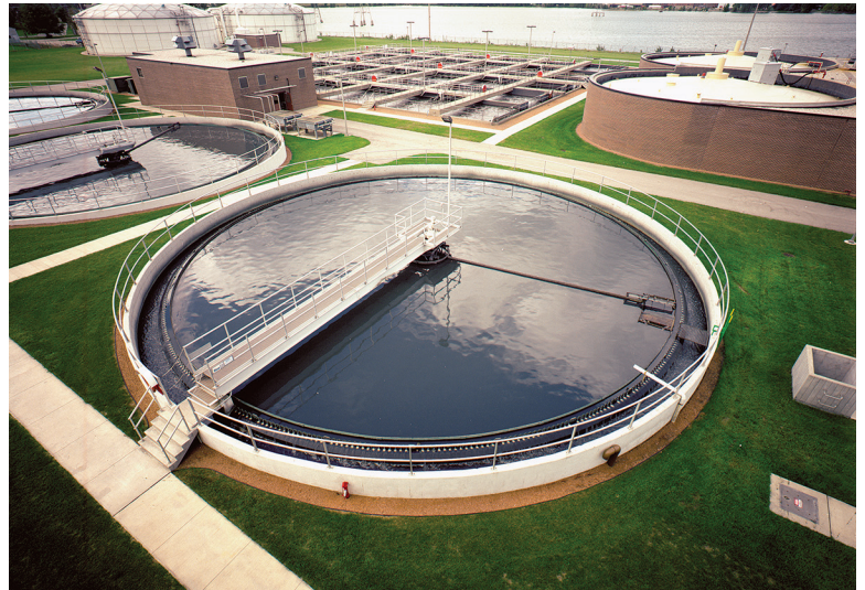
Between corrosion, maintenance, and changes in flow, keeping a clarifier working at peak performance can be challenging. Complimentary inspection by OEMs for circular or rectangular clarifiers help assess equipment condition and performance. (Tow-Bro clarifier from Evoqua Water Technologies)
