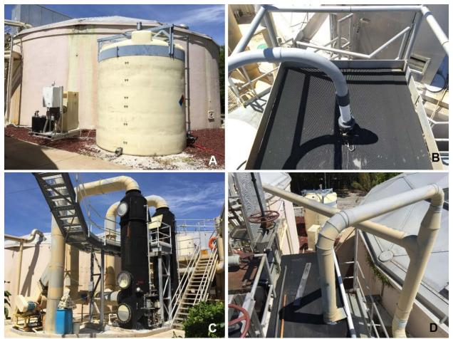
Figure 3 – Calcium Hydroxide Slurry System at the Siesta Key WWTP A) Feed system and storage tank, B) Chemical discharge line, C) Odor control scrubbers, D) Odor control scrubber draw points.
