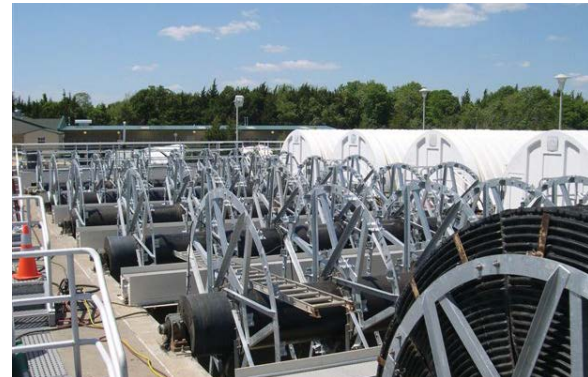
Media & Support Structure Replacement
